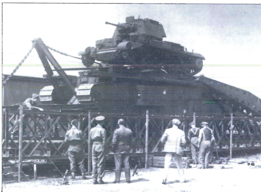
A double/single Bailey Bridge under test load at Christchurch, in early 1941. Donald Bailey is in the foreground in his familiar sports jacket and cap.
