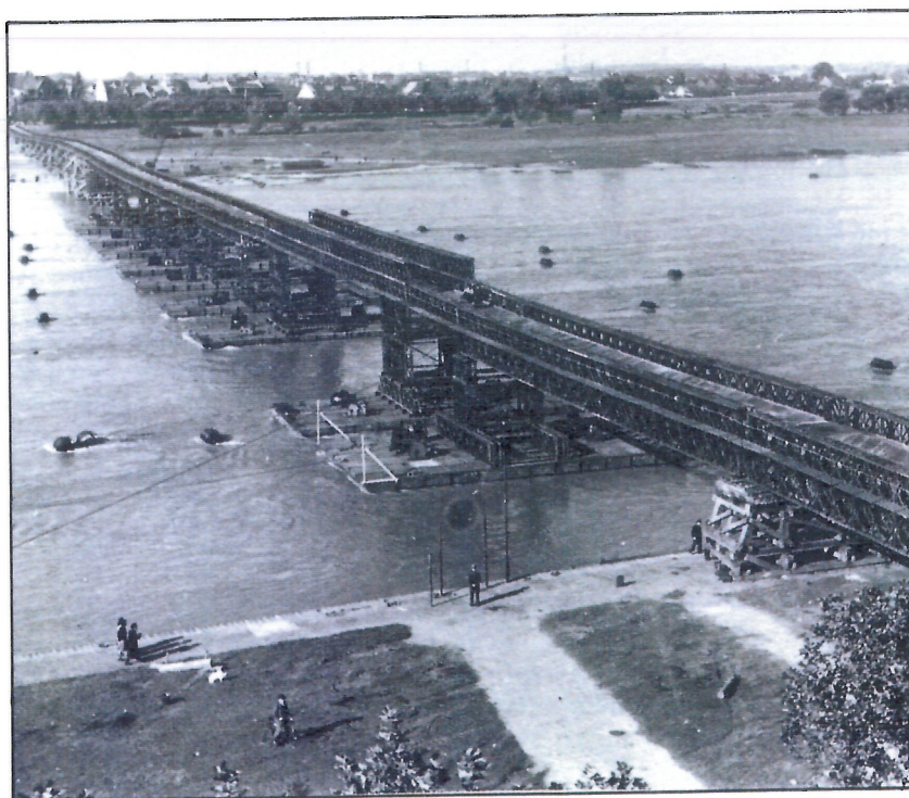
Freeman Bridge was one of the semi-permanent Rhine bridges built after the War. The Class 24 bridge was built at Dusseldorf in two months; its length was 2391ft overall and it was opened to traffic in October 1945.
