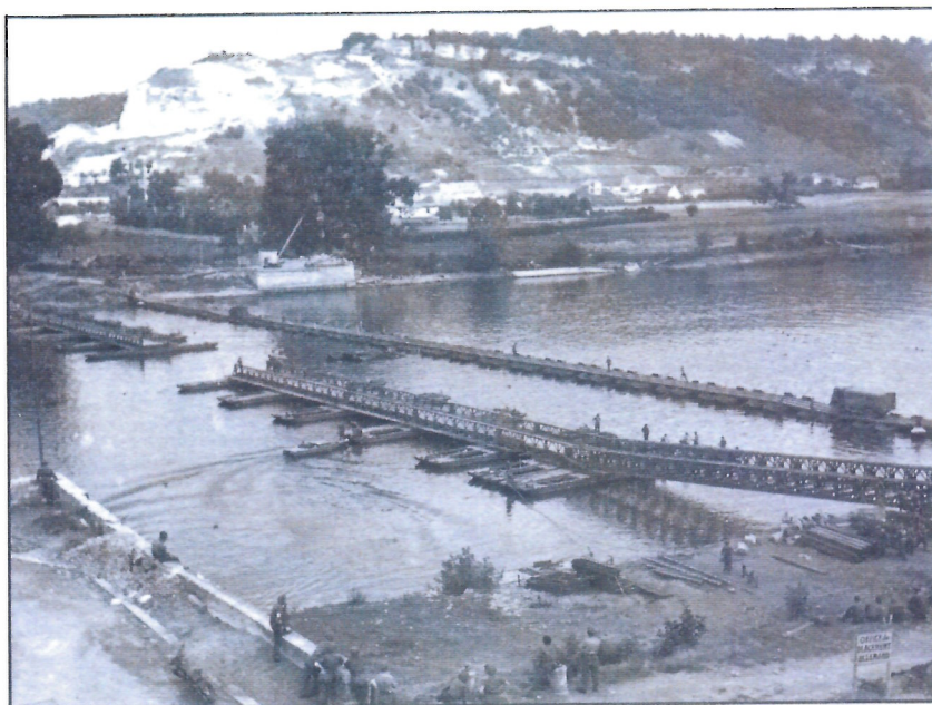
The David and Goliath Bridges built across the River Seine, at Vernon, France. The 694ft Goliath Class 40 Bailey was built on 26-27 August 1944 by 7 Army Troops Engineers; David Bridge is a Class 9 Folding Boat Bridge.
