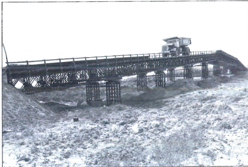
A Bailey Bridge from Thos. Storey (Engineers) used for construction equipment access on a site in the UK.
