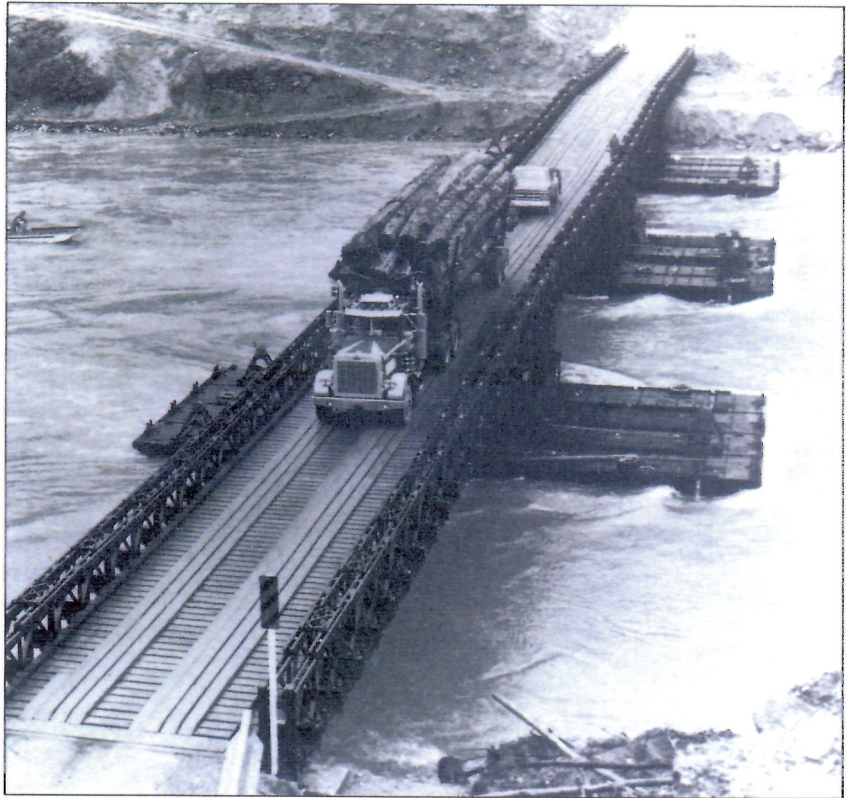
Here, an Acrow Panel Bridge is supported on Storey Uniflote pontoons to provide a floating bridge for the logging industry at Revelstoke, British Columbia, Canada.
