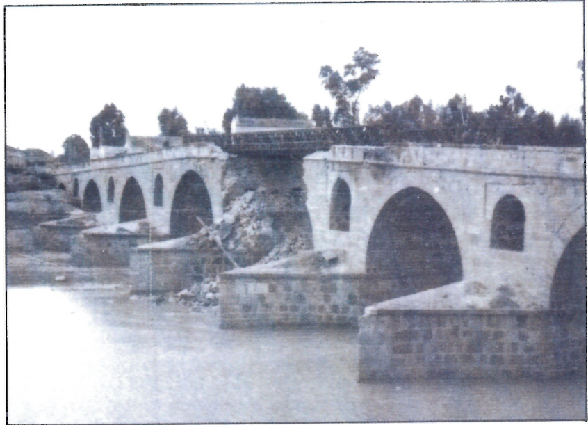
The first ever operational Bailey Bridge, a 100ft triplelsingle, built across the River Medjerda at Medjez el Bab, Tunisia, during the night of 26 November 1942.
