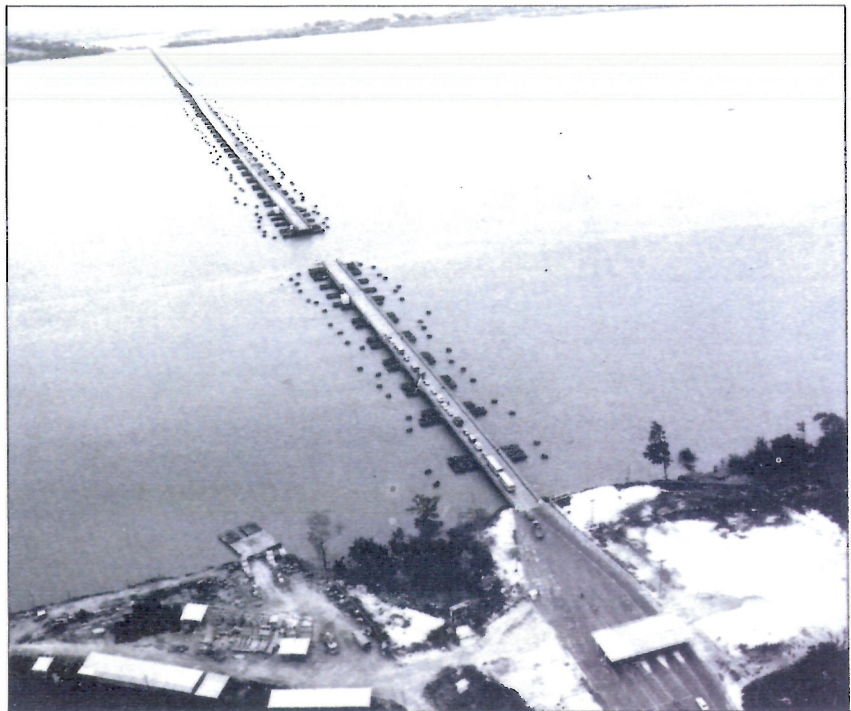
This double lane floating Acrow Panel Bridge crosses the Demerara River in Guyana. At just under 2km in length, it is one of the longest floating bridges in the world and features a retracting span to allow passage of ships. Thos. Storey (Engineers) completed its construction in one year.
